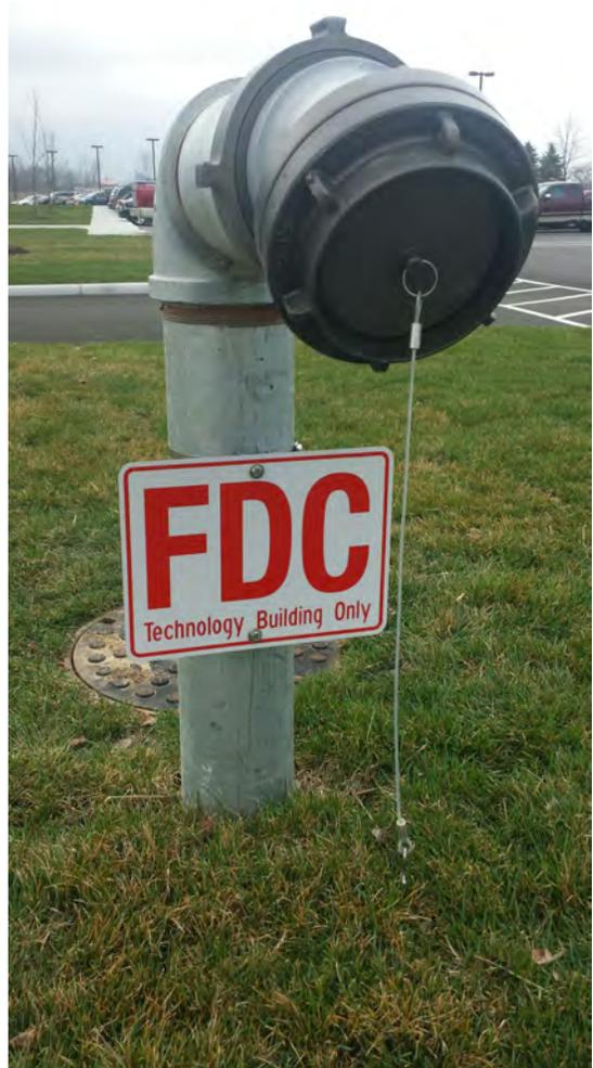
*Photo shows a correct FDC, except that the piping up to the 45 degree adapter should have been painted OSHA Safety Red*
